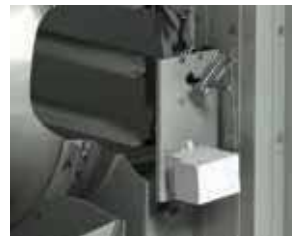
Isolation Damper and Actuator
